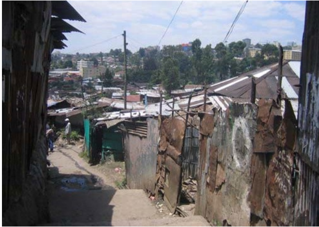
Plate 5: Informal dwelling in informal settlements
